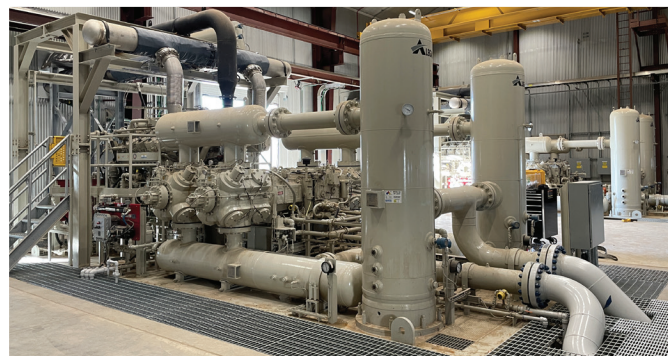
North Branch Unit 7 - Waukesha L7044/Ariel KRK/4 Reciprocating Engine-Compressor Package
