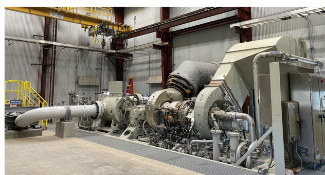
North Branch Unit 5 - Solar Centaur 40 Turbine-Compressor Package
